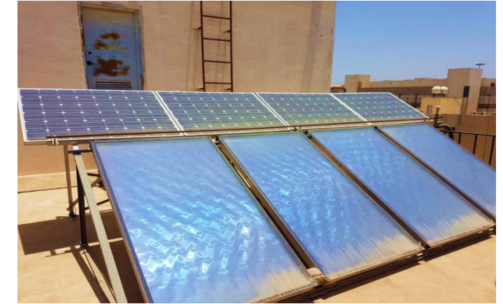
PV system 8 PV panels assembled in parallel- peak capacity 1.480 kW peak Electric batteries DC/AC inverter Solar collector system 8 flat plate collectors arranged in a series: parallel (4:2) configuration- total effective area 20 m 2 Heat exchanger: 16 kW.
