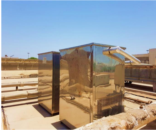
Thermal sink system 2 water cooling units, capacity of cold water tank 500 l, compressor H.P : 2.5, cooling capacity : 1000 liters/h. Heat exchanger: 9 kW
